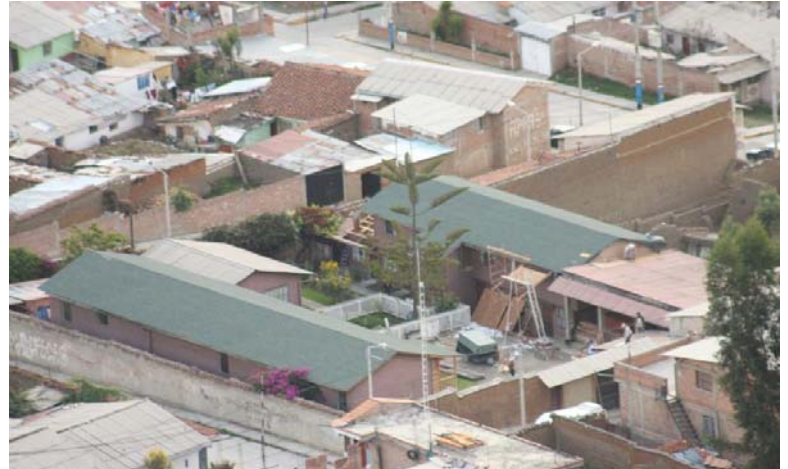
Training Center Roofing Project
