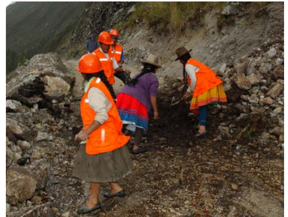
Clearing rock slide
